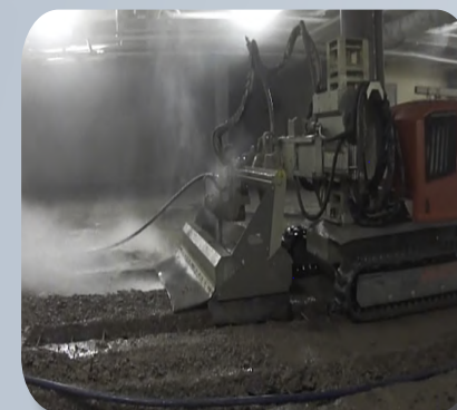
Demolition of Concrete by Robotic Method and Hydro Cold Cutting Method
