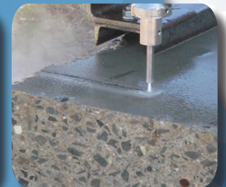
Demolition of Concrete by Robotic Method and Hydro Cold Cutting Method
