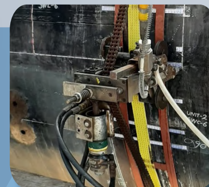
Hydro Cold Cutting and Decommissioning of Flammable Vessels/ Columns by Hydro Cold Cutting
