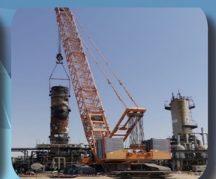
Hydro Cold Cutting and Decommissioning of Flammable Vessels/ Columns by Hydro Cold Cutting
