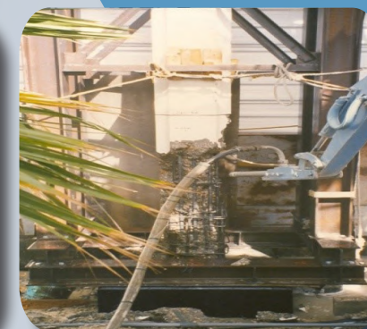
Demolition of Concrete by Robotic Method and Hydro Cold Cutting Method
